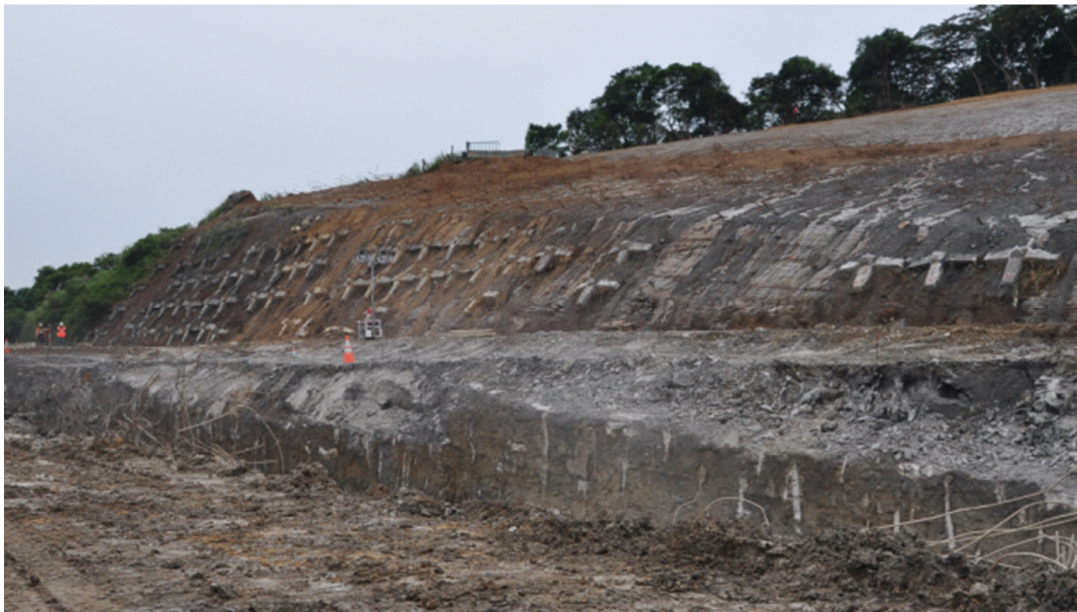
Figure 7. Anchors that were completely intact below the sliding failure plane
