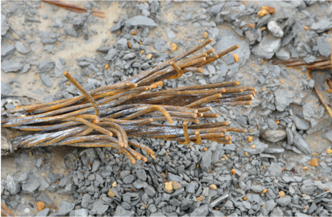
Figure 6. Test anchors remaining on the sliding failure plane
