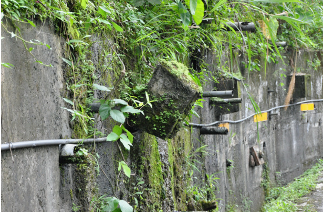
Figure 15. Damage of the anchor head induced by the breaking of the free length
