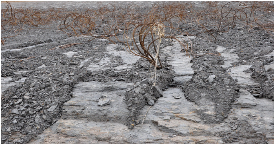
(b) Lower part of the sliding failure plane (the deployed anchors have been pulled off)
