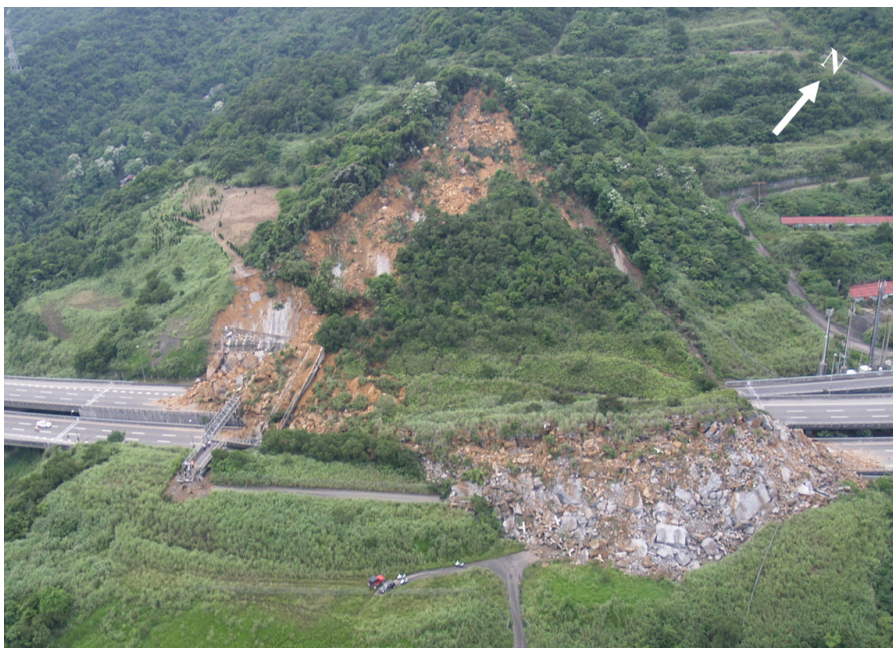
(c) Photographed from the southeast to the northwest (Taiwan Geotechnical Society, 2011)
