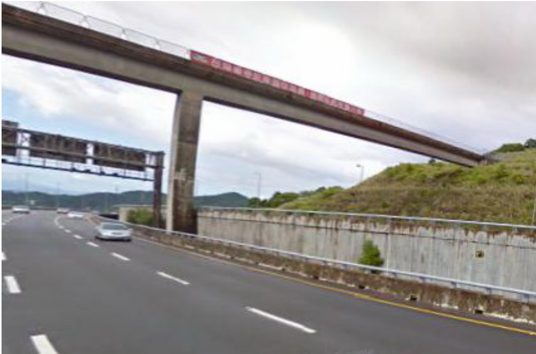
Figure 10. Bending deformation and cracking on the pier (Google Earth, 2010)
