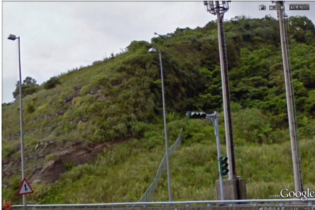
(a) Before overlaying
