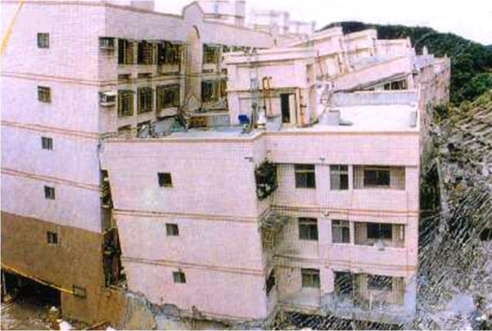
Figure 1. Lincoln County anchor block slope disaster (New Taipei City Government, 1997)
