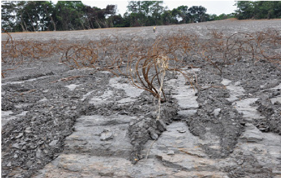
Figure 3. The rusted snapped anchors remaining on the sliding failure plane
