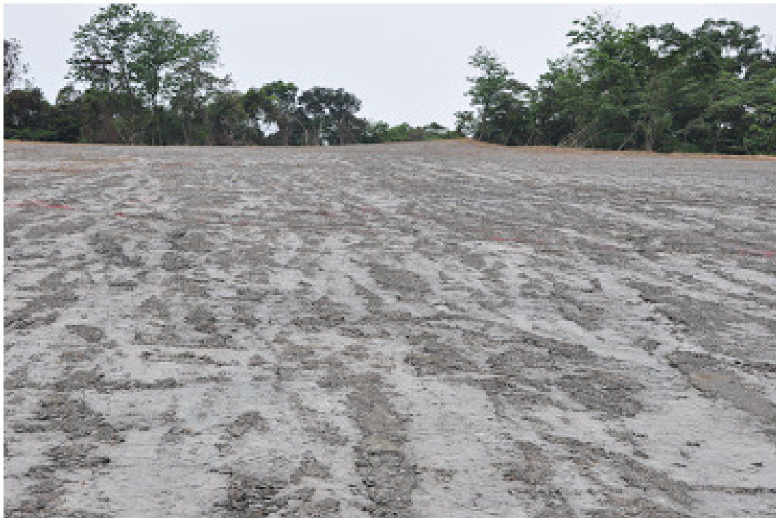
(a) Upper part of the sliding failure plane (no anchor deployed)
