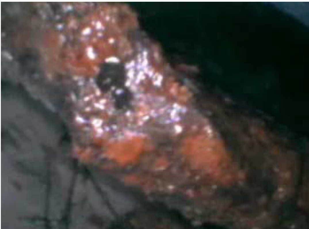
(c) The anchor affected by groundwater
